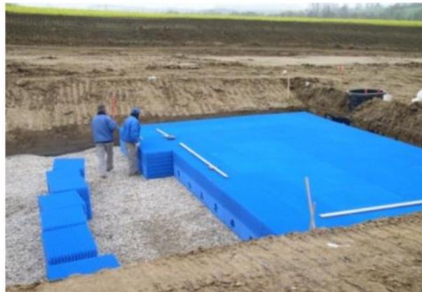
Setup of an infiltration trench with filling
