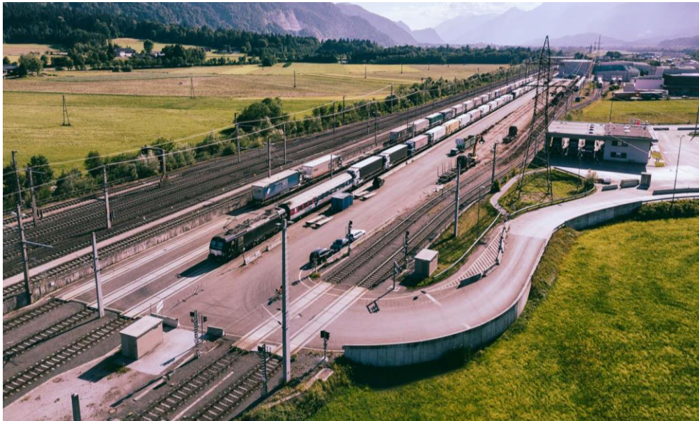
Figure 11. Rail Freight Centre Wörgl
