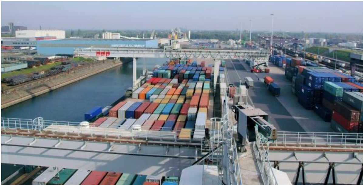
Figure 17. STS quay cranes in trimodal river terminal Source: ect.nl/en/terminals/hutchison-ports-duisburg
