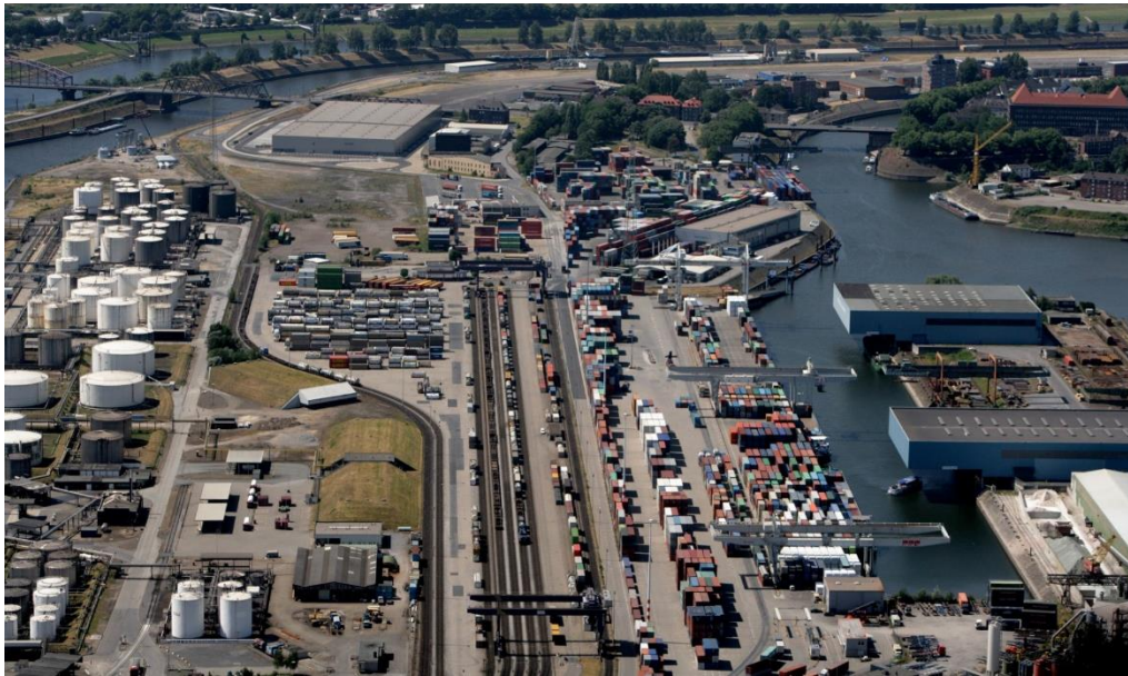
Figure 7. DeCeTe Duisburg Terminal
