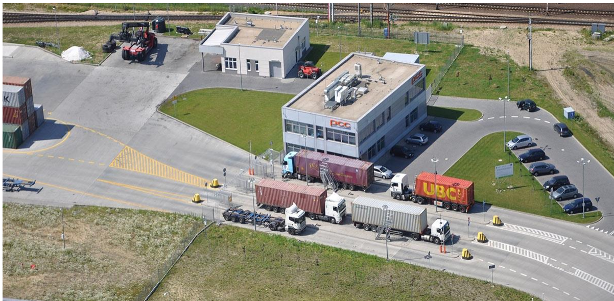
Figure 47. Semi-automatic identification at the gate of rail-road terminal
