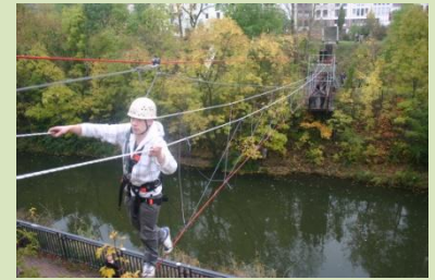
Building a bridge over the canal
