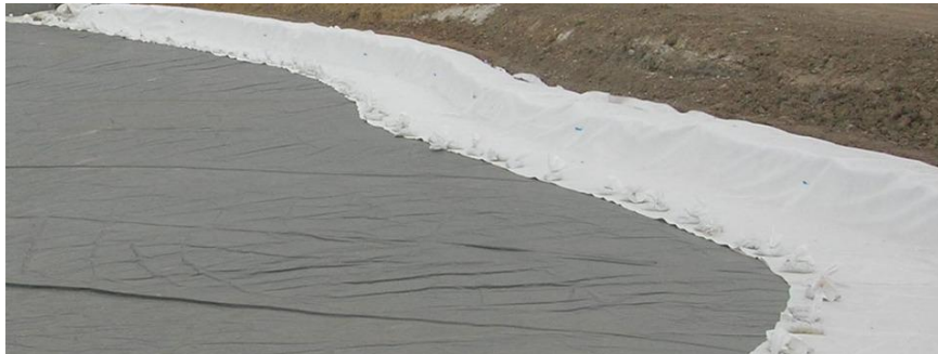
Geosynthetic Technology Ltd Landfill Lining & Capping
